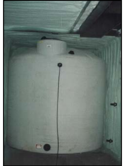
Storage tank (2100 gal. shown) and salt loading chute (brine maker removed)
