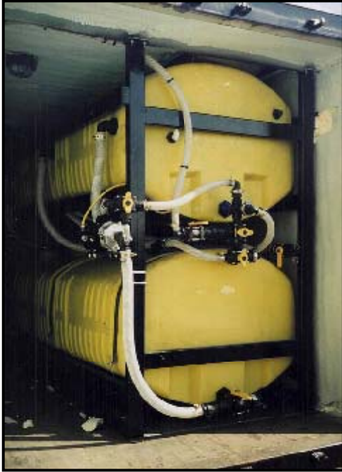
Brine making unit 1000 or 750 gal. polyethylene tanks Steel containment frame with corrosion resistant coating. Stainless option. Stainless and poly. plumbing components
